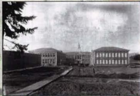
1915 photograph during construction of Franklin High School, looking north.
